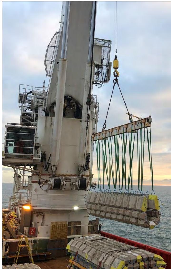
Figure B.6 – Concrete Mattress Installation
